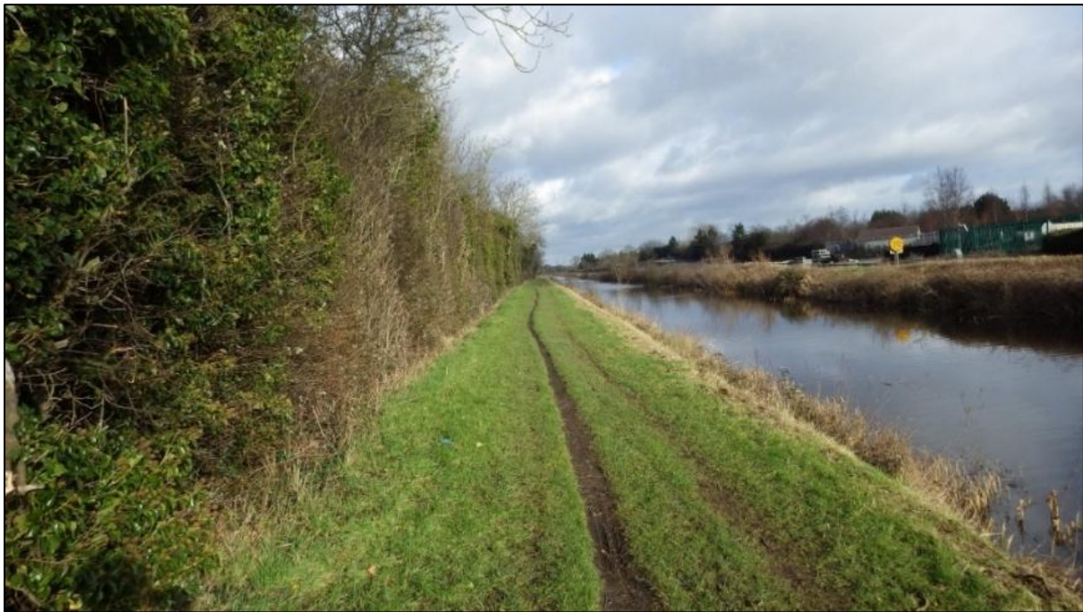
Figure 2-2 Existing Towpath between Collins & Pakenham Bridges
