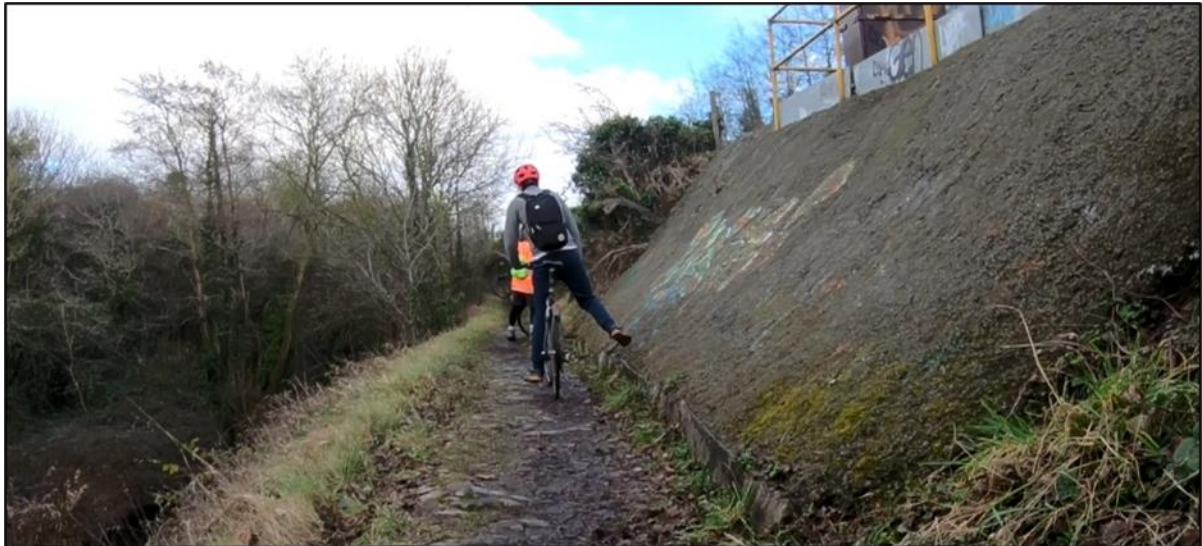
Figure 2-5 Pinch point between towpath and the railway signal
